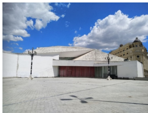
Figure 6. Various angles at this building
